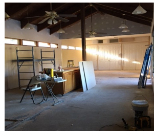
Walls ready for finish!
