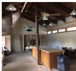
Sheet rock going up.
