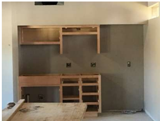
Kitchen Cabinetry going in.
